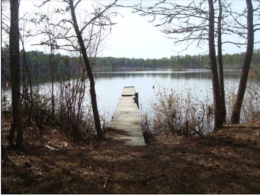
Figure 11. A pier extends west into Little Muddy Lake from the southern part of the dam. The pier is either a modern replacement or later addition, ca. 1980s–1990s.
