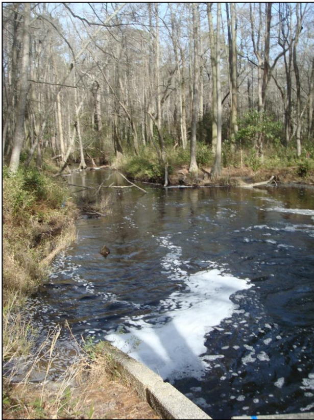
Figure 12. Downstream view of Big Muddy Creek from the dam embankment above the spillway outlet.
